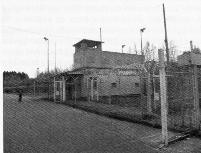
Main entrance hardened control point.
